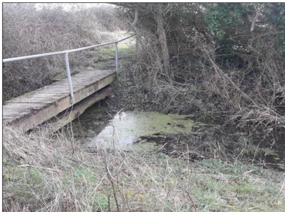
View 3: Orsett Fen Sewer (ref. F)
