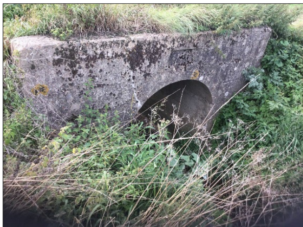
View 6: Golden Bridge Sewer (ref. G)
